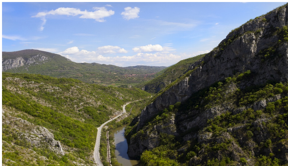
View of non-electrified railway track (as well as two-lane road) in Sićevo Gorge, on Corridor Xc, Serbia.
