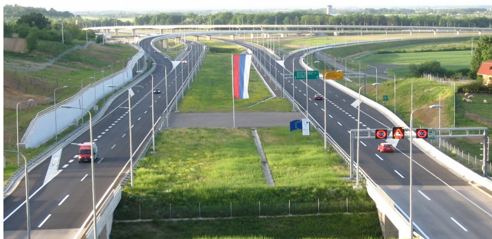
Newly built Mahovljani Interchange on the Banja Luka – Dobož motorway in Bosnia and Herzegovina.
