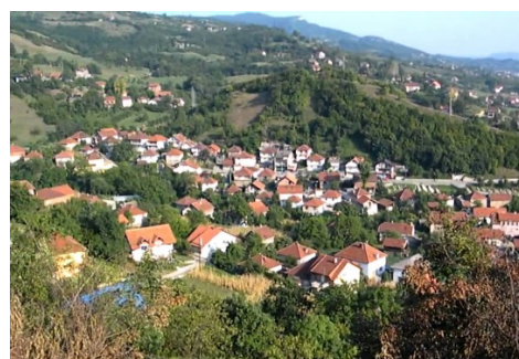
Aerial view of Donja Gračanica in Bosnia and Herzegovina.
